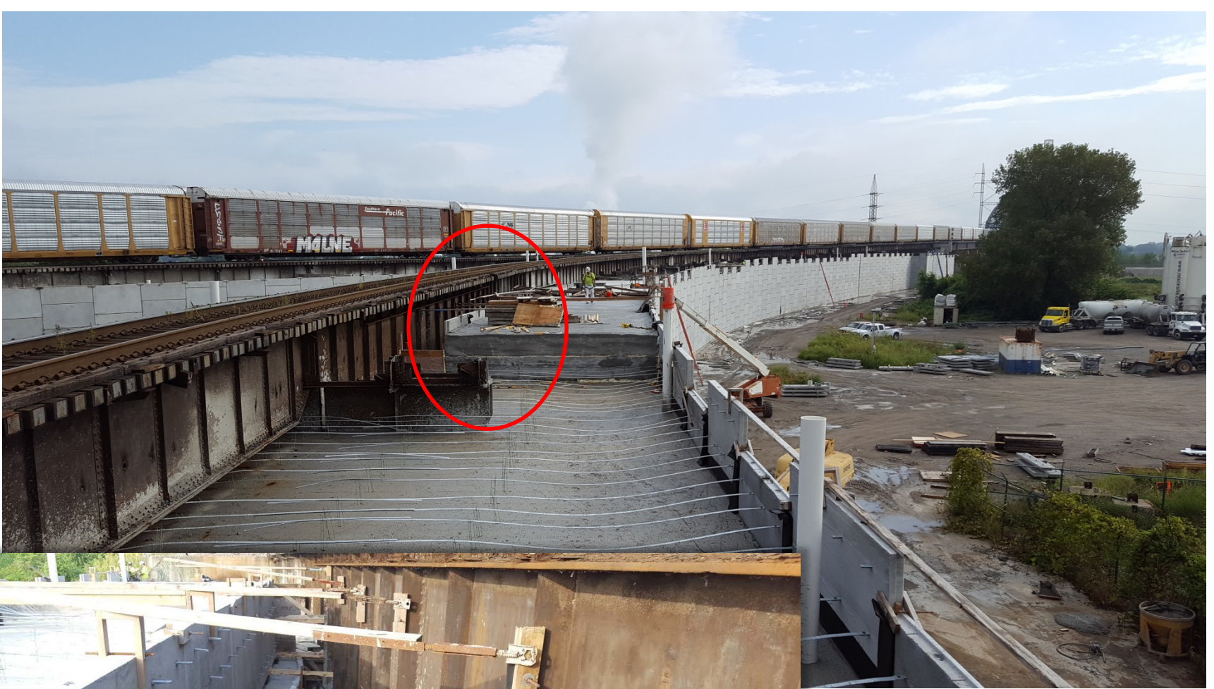
LCC Placement Ferry Street Bridge
