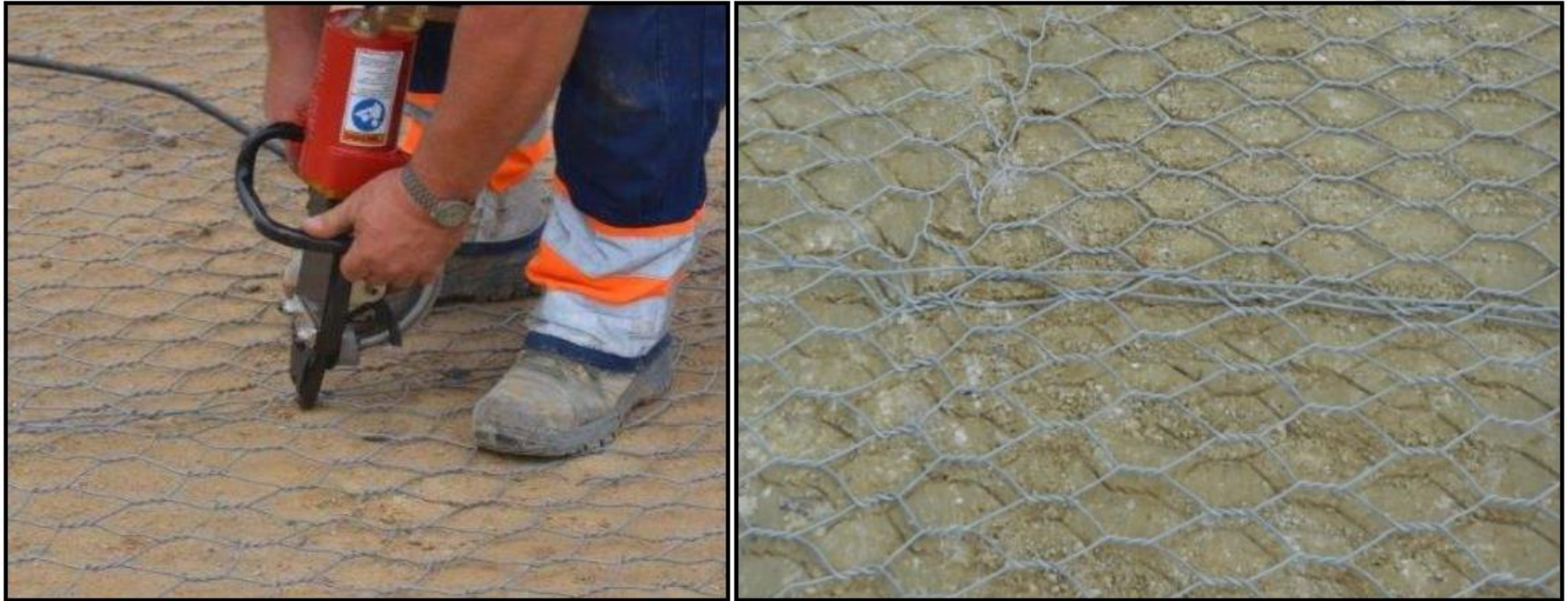
Fig. 10 – Placing of rings by pneumatic lacing gun to connect two adjacent wire mesh tails
