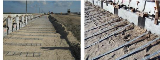
Figure 17, Metallic Reinforcement (Inextensible). Left: metallic grid. Right: Ribbed Strips.
