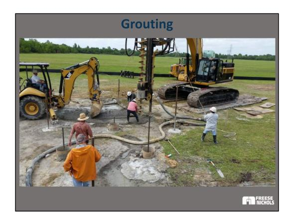
The foreman watches carefully to be sure the auger is not raised too fast, which could allow soil to enter the pile.
