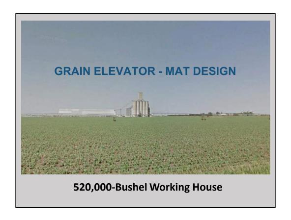
A Farmer's Cooperative in Nebraska planned a new grain storage and handling facility along the railroad tracks. It would be a slip-formed concrete grain elevator consisting of ten cylindrical cells about 137 feet tall, arranged in two rows. The structure would be a "working house", meaning that it would include a vertical bucket elevator called an "elevating leg".
