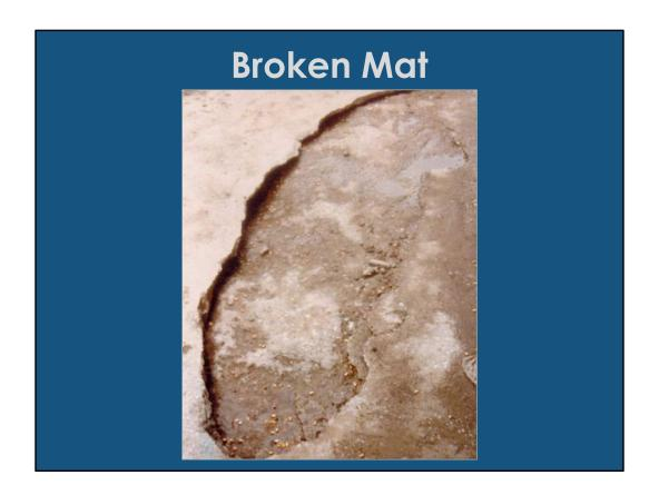
In the spring, when most of the grain had been removed through normal seasonal operations, the builder uncovered the foundation. The cantilever had sheared off.
