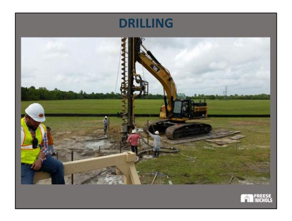
Augered piles are installed by drilling with a hollow-stem auger. The opening at the bottom of the auger is plugged with a cork. When the desire depth is reached, the grout pump is started, the auger is raised a few inches to make room for the cork to be expelled, and the grout is pumped to fill the hole as the auger is slowly withdrawn.
