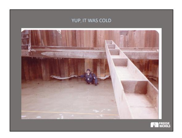
I swept the bottom with my hand while following a pipe across the excavation. The pipe was moved, and the procedure was repeated until the entire surface had been examined. Footing corners were marked using a plumb pipe, and I confirmed that the entire bearing surface was ready
