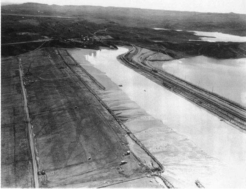
Fort Peck Dam
