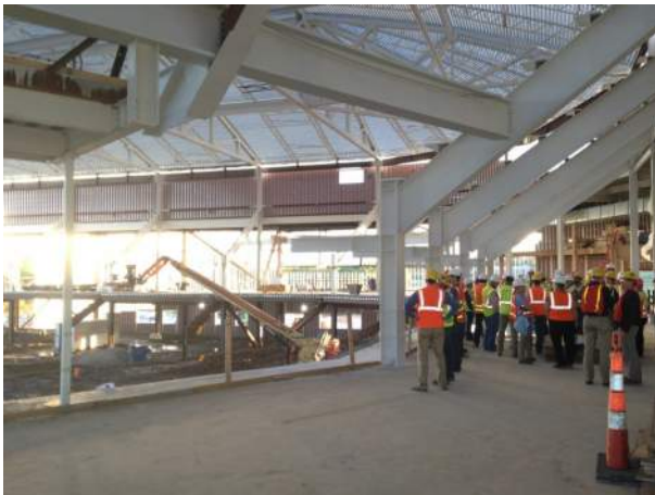
UNO Community Arena Site Tour
