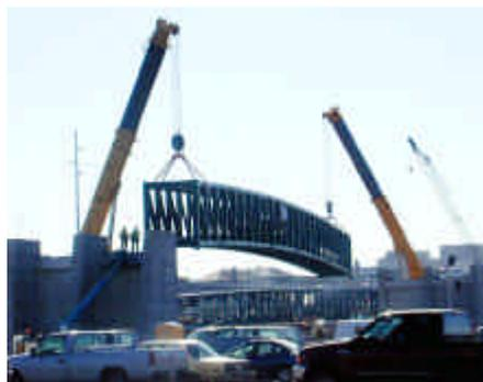
meetings with railroad officials, Federal, State, and City representatives resulted in a 264 foot clear span over the tracks. This is the longest span through truss that could be designed using commercially available rolled steel tube sections.
